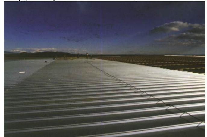
▲Newer-generation metallic coatings have led metal roofing into very low-slope applications, which compete with traditional flat-roof alternatives.
