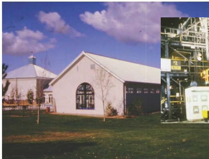
▲ Advances in metallic coatings have expanded the applications for the use of steel in roofing (above). Coatings (right) are applied in a continuous hot-dip line at the producing mill.
