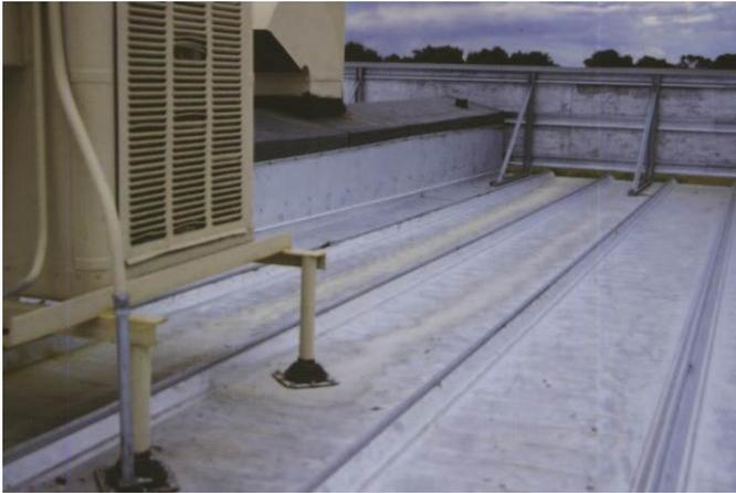
Drippage from a rooftop unit can cause corrosion as shown on this 1 ½-year-old roof. In another year and a half, the white zinc oxide trails will turn red with iron oxide.
