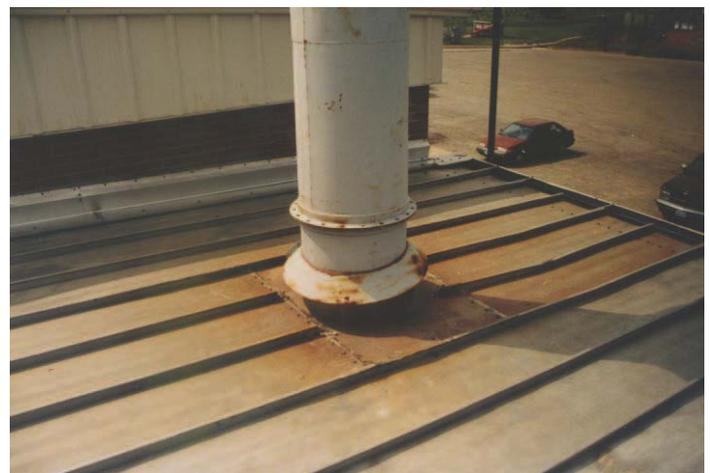
▲Exhaust flues that discharge gases from burning fossil fuels can cause a micro-acid rain environment near the flue.
