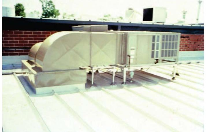
▲ This frame-mounted HVAC unit uses pipe supports that extend to the building structure and are flashed through the roof using rubber pipe flashings.
