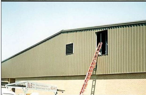
Figure 20-12 Retrofit Endwall Installation
