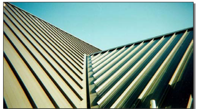
Figure 4-20 The Terms Hydrokinetic Roof, Steep Roof, and Architectural Roof Are Often Used Interchangeably
