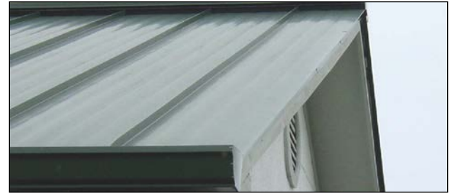
Figure 4-17 Architectural Panel Roof System
