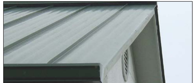
Figure 4-17 Architectural Panel Roof System
