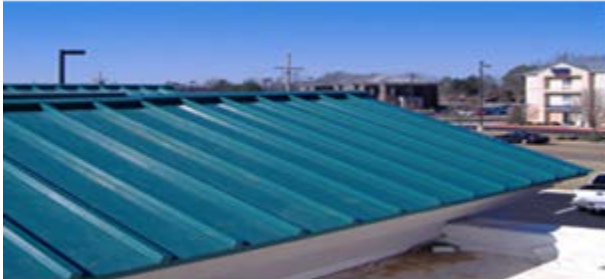
Figure 4-9 Modern Batten Style Roof
