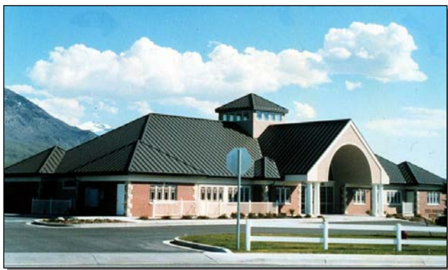
Figure 4-3 Vertical Roof Panel Installation
