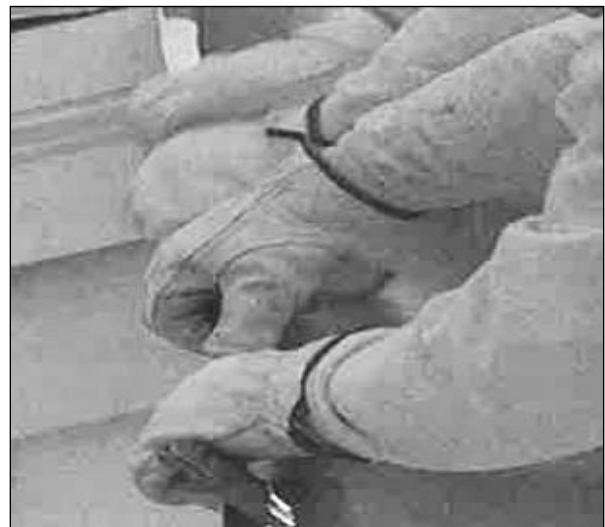
Figure 9-6 Gloves Offer Protection to the Hands and to the Roof Panel.
