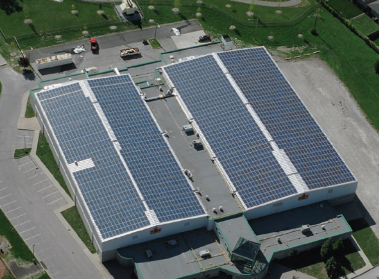
Tecumseh Arena, in Tecumseh, Ontario, holds what is currently the largest operating rooftop solar PV system in Canada. The 508-kW DC system consists of 2212 230-W panels, two 250-kW inverters, and more than 6000 mini clamps and PV kits.
