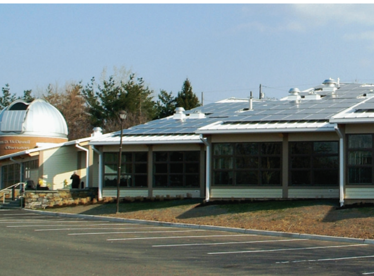
New Jersey Meadowlands Commission's Center for Environmental and Scientific Education's 165-unit rooftop crystalline solar panel array generates electricity for the building's power needs. The solar units are expected to produce a peak maximum of 33,000 watts of electricity.
