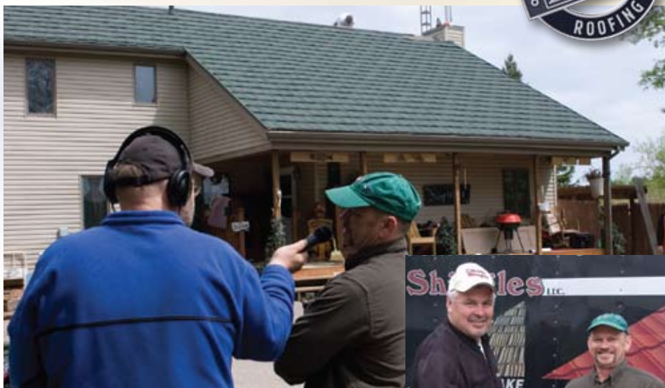
Vince Marik is interviewed as he views the new Investment Grade Roof being installed on the home he shares with his wife and seven children.
