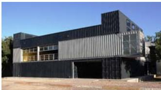
The Student Center at Monterrey Technical University utilizes a unique approach to recycling. The colorful open structure uses standard 40-foot recycled steel containers
