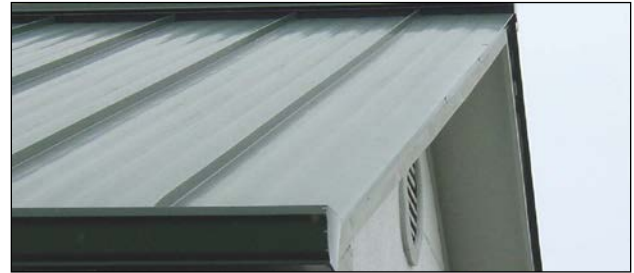
Figure 4-17 Architectural Panel Roof System
