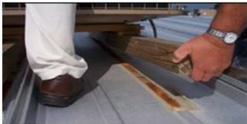
Figure 3. Roof corrosion from treated wood
