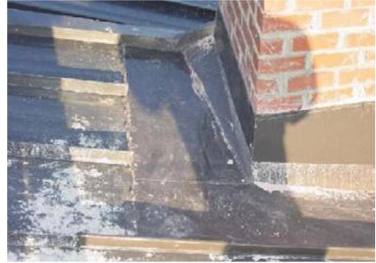
Figure 4. Cement, mortar, and related products can damage metal roofs
