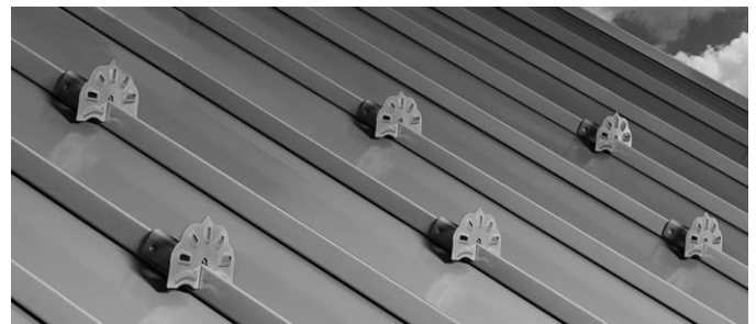
Figure 8B: “Cleave” type snowguard system
