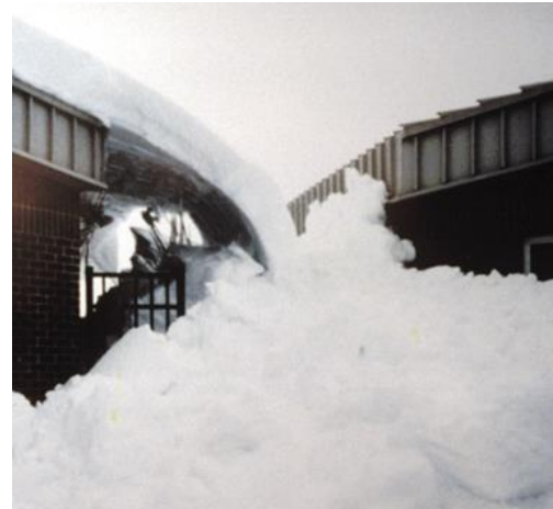
Figure 5: Sudden release of roof snow
