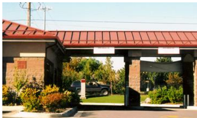
Fig. 7: De-icification cabling integrated with snow
