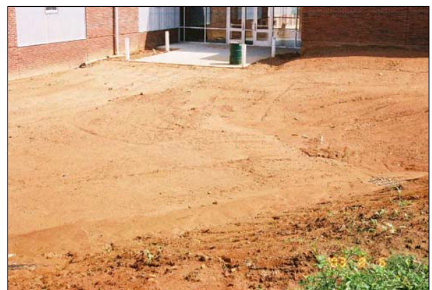
Figure 11-15 An Impossible Situation (Eliminating Dirt From Construction Sites)
