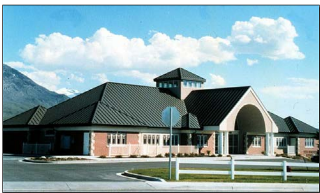
Figure 4-3 Vertical Roof Panel Installation
