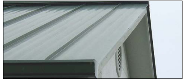
Figure 4-17 Architectural Panel Roof System
