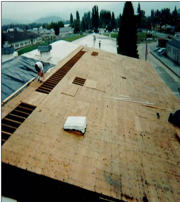
Figure 6-6 A Plywood Solid Roof Deck Substrate
