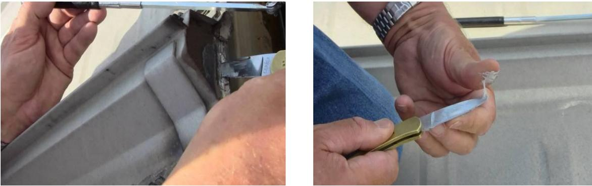
Figure 14 – Eave closure probed with knife edge (left) produced a sample of the butyl sealant that exhibited
