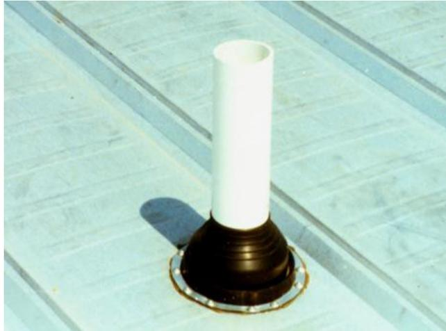
Figure 2 – Best-practice flashing of round roof penetration.
