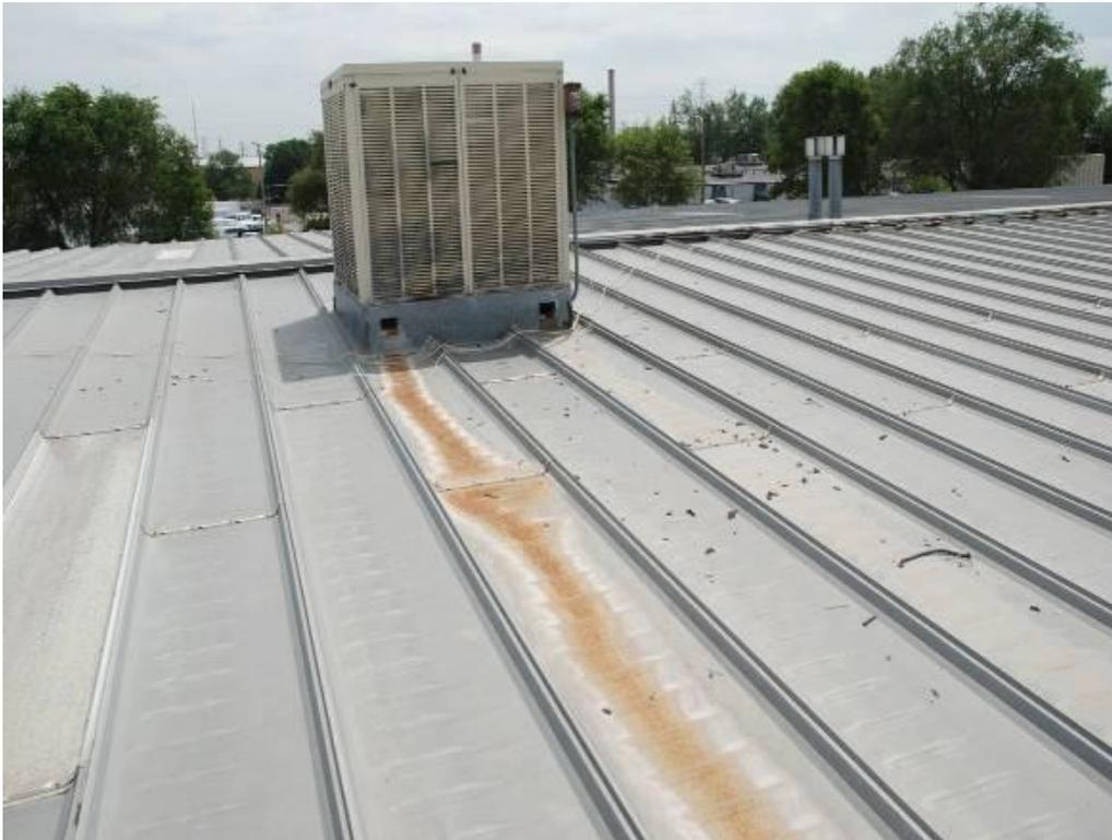
Figure 20 – Accelerated corrosion of 55% Al/Zn sheet due to improper drainage of copper ion-containing HVAC condensate.
