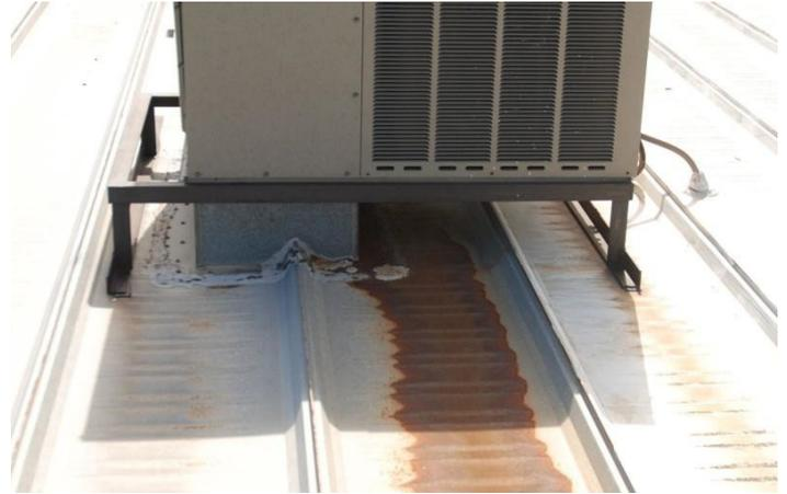
Figure 21 – Typical examples of poor HVAC mounting
