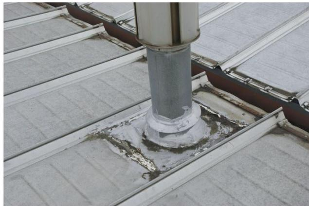
Figure 19 – Two examples of flashing round penetrations
