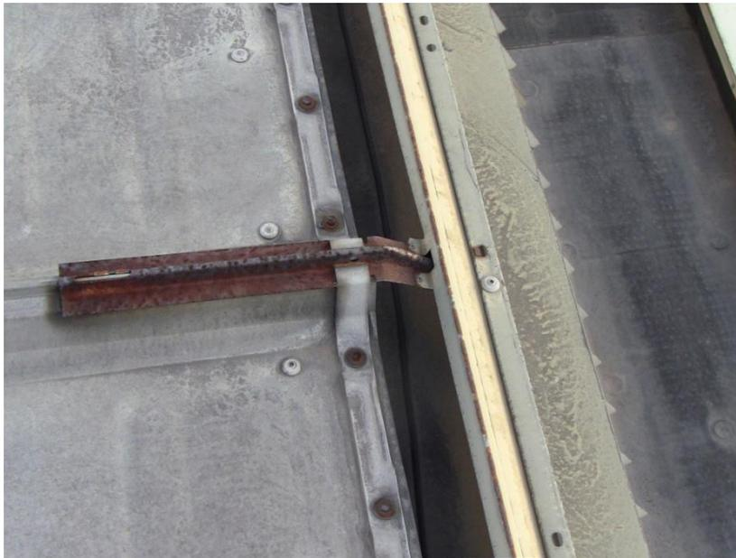
Figure 23 – Gutter hanger performance of galvanized G-90 steel after 32 years in Ohio.
