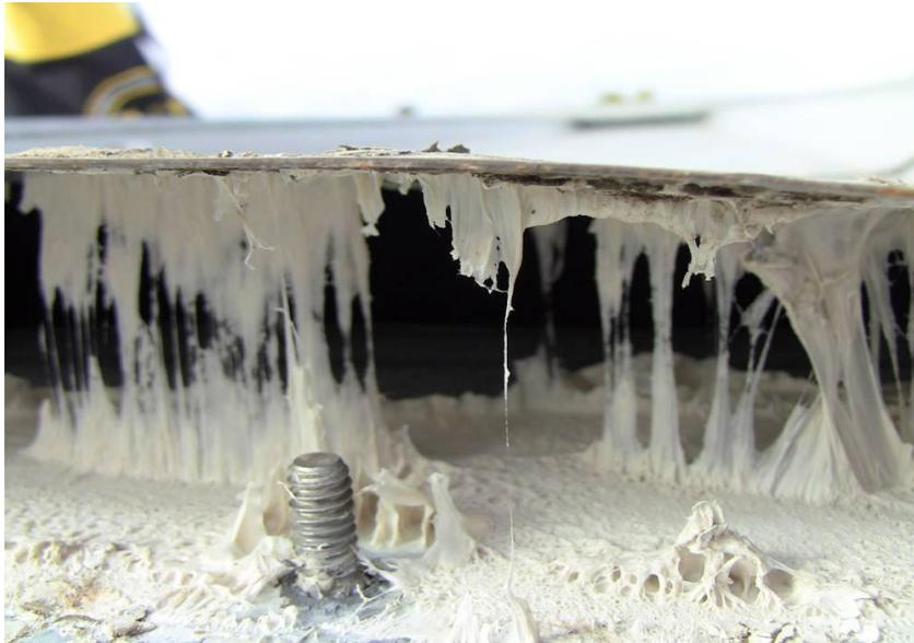
Figure 13 - Excellent elasticity demonstrated by the butyl sealant on the Denver roof after 33 years.
