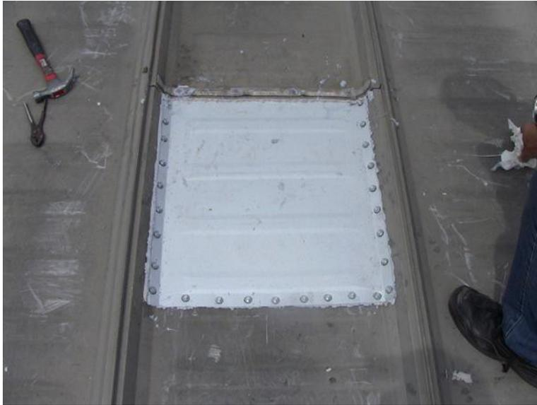
Figure 9 – Completed patch after removal of exposed sample.
